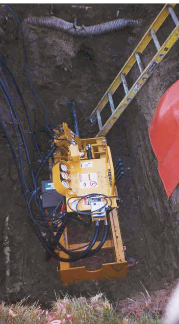
Pit-launch HDD units are now being used on FFTP jobsites with extremely limited space.
